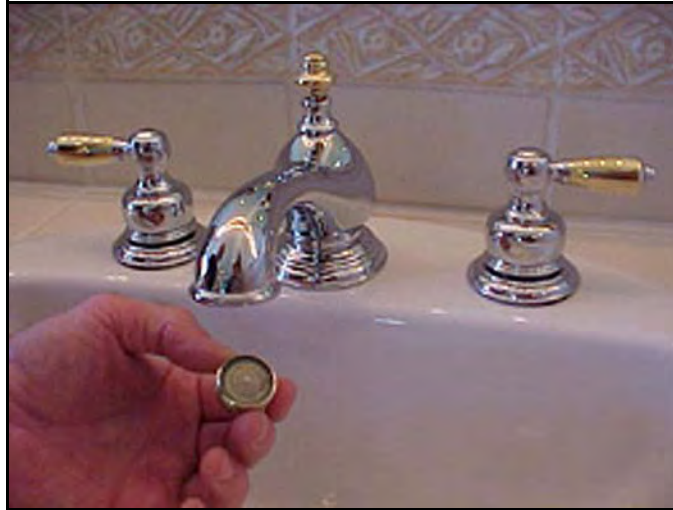
Remove the Aerator Screen to Repair Blockages
