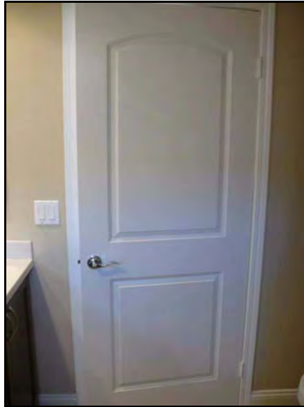
Interior Wood Door
