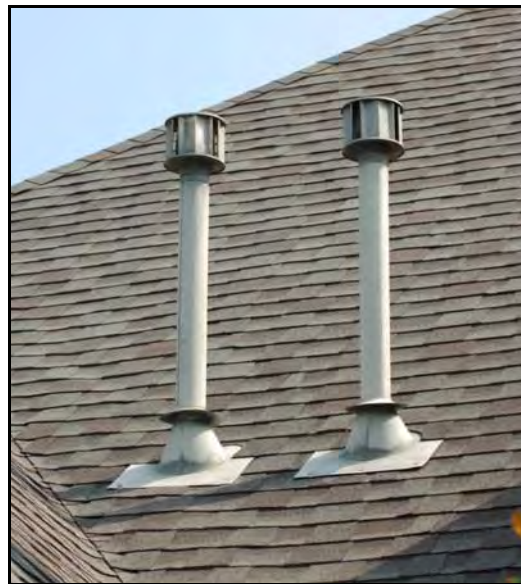
Example of roof penetration flashing
