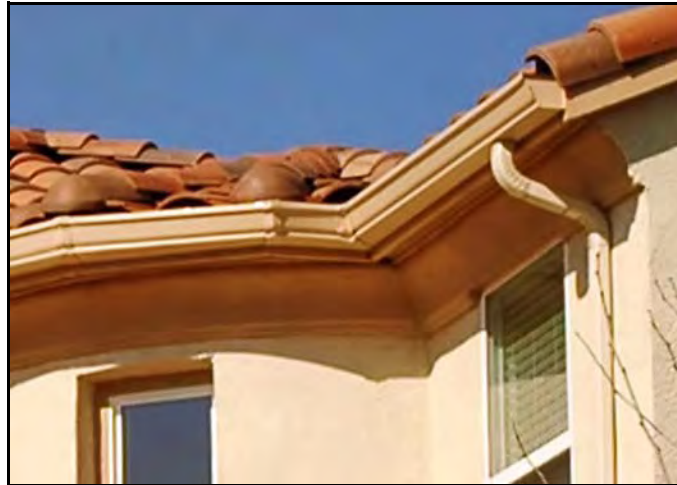
Gutter and Downspout
