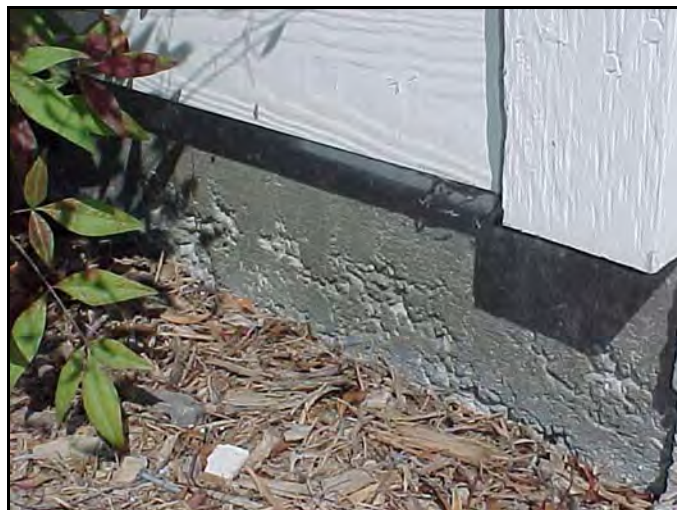
Slab on Grade Foundation
