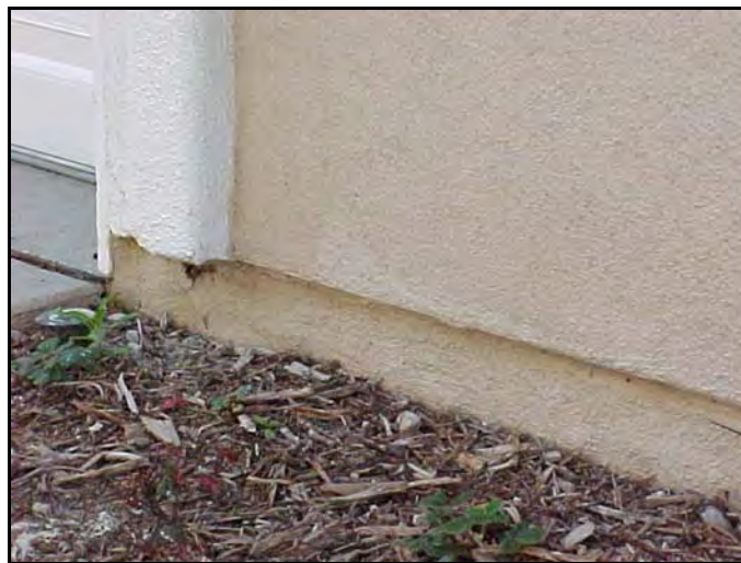
Base of Exterior Wall Finish
