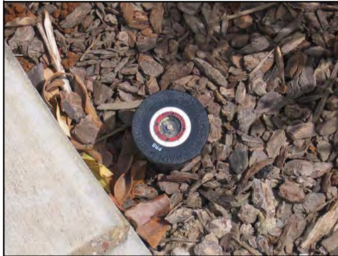
Irrigation Sprinkler Head
