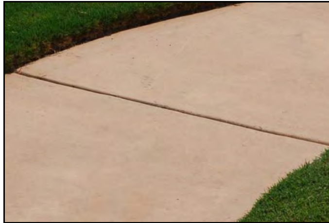
Expansion Joint in Concrete Walkway
